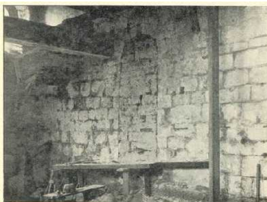
DOGWAY IN NORTH WALL OF CHURCH.
