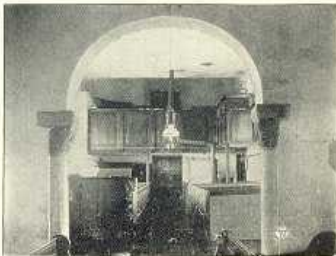
INTERIOR FROM ALTAR LOOKING W. (BEFORE RESTORATION).
