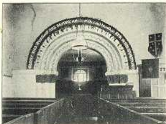
INTERIOR LOOKING EAST (BEFORE RESTORATION).
