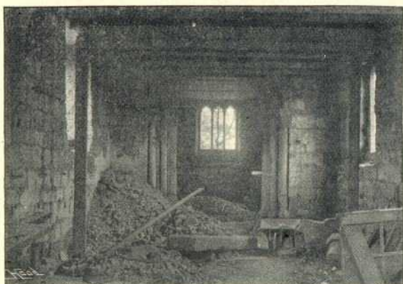
INTERIOR LOOKING EAST (DURING RESTORATION).
