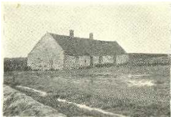
EXTERIOR VIEW OF BUILDING.
