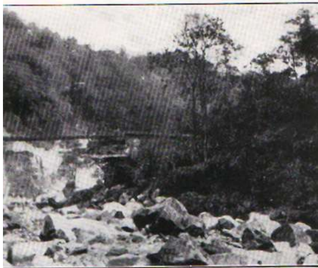
RAILWAY BRIDGE IN ARNCLIFFE WOODS AFTER FLOOD IN JULY, 1930.
