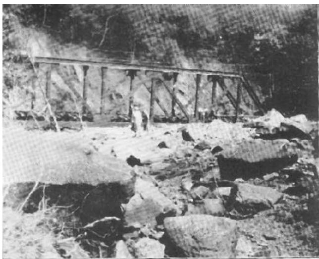
NEW RAILWAY BRIDGE IN ARNCLIFFE WOODS, AS DESTROYED BY THE FLOODS IN SEPT., 1931.
